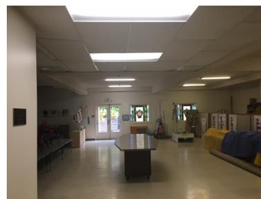
Gary Schick has replaced all of the incandescent lighting in Young-Wheeler Hall with LED lighting. He also replaced the old and cracked and faded lenses with new lenses. He previously installed
